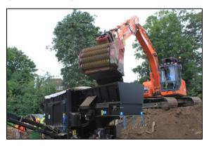
Photo 2 - Loading the Xtract machine for on-site processing of knotweed infested soils
