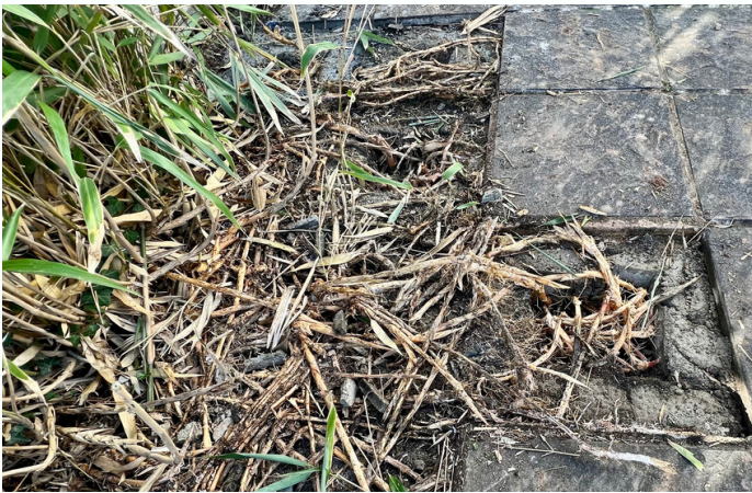
Running bamboo spreading underneath patio slabs
