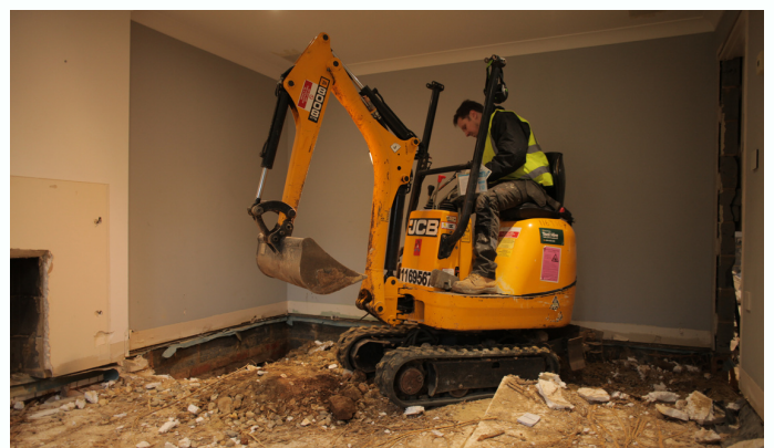
Excavation of bamboo beneath living room floor
